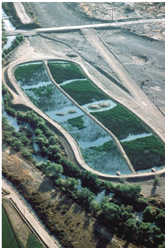
The Cobble Site Demonstration Treatment Wetland for the city of Phoenix tests the feasibility of recreating habitat in the dry channel of the Salt River.
