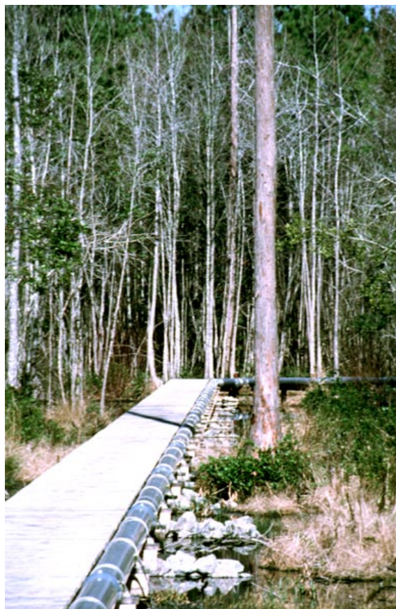
Gated pipes on raised boardwalks allow access to more than 600 acres of treatment area in the Vereen Natural Treatment Wetland in South Carolina.
