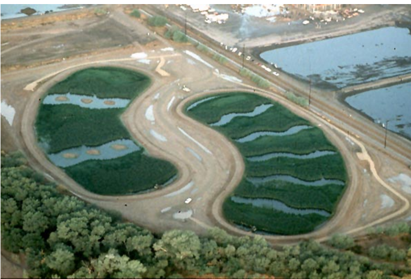
The Hayfield Site demonstration wetland at Tres Rios west of Phoenix, Arizona, includes two cells with variable numbers of deep water zones to test their effect on hydraulic efficiency and wildlife habitat.
