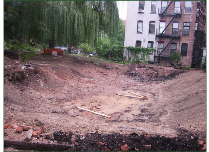
The pond as excavated, prior to liner installation.
